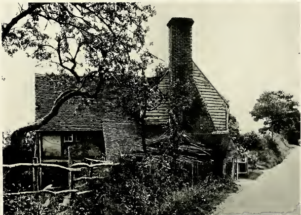
FARMHOUSE NEAR MARDEN ( Upper ) OLD FARMHOUSE NEAR COWBEECH ( Lower )
